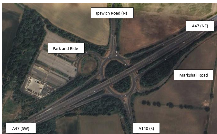
Image 7.1 A47 Norwich Southern Bypass/ A140 Ipswich Rd grade-separated roundabout
