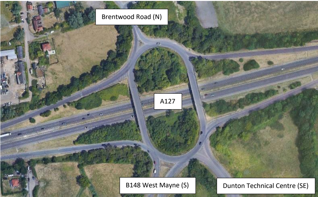
Image 7.21 A127 Southend Arterial Rd / B148 West Mayne roundabout
