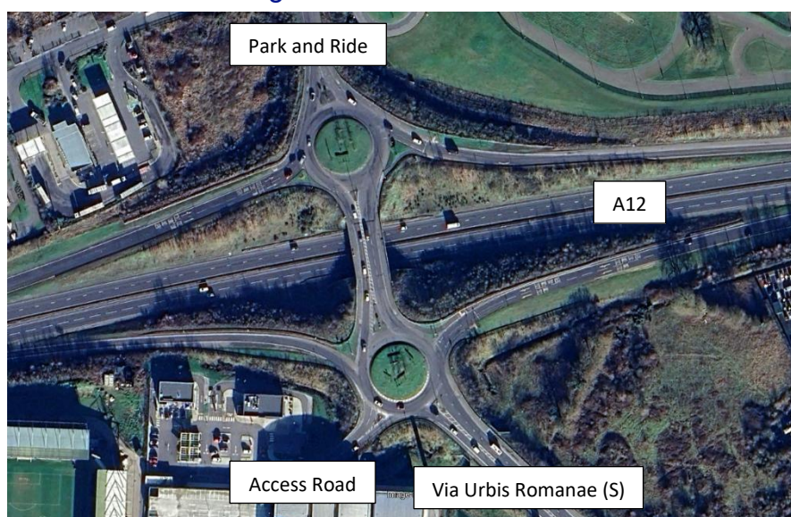
Image 7.14 A12 Severalls Interchange
