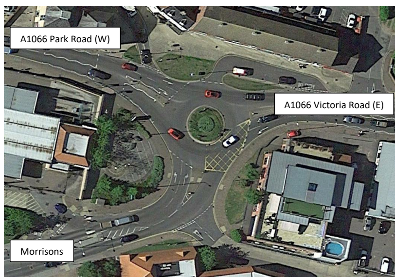
Image 7.30 A1066 Victoria Rd / Morrisons access roundabout
