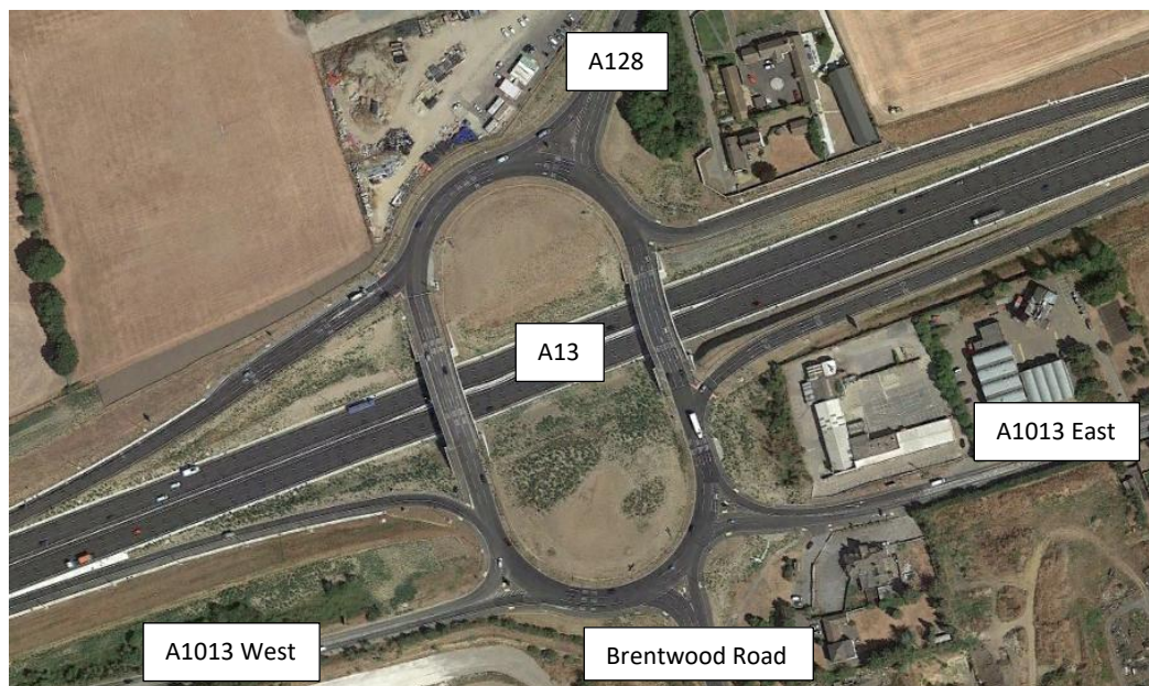
Image 7.23 Orsett Cock A13 Stanford le Hope Bypass / A1013 Stanford
