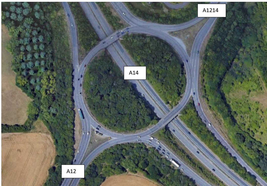
Image 7.6 A14 J55 Copdock Interchange
